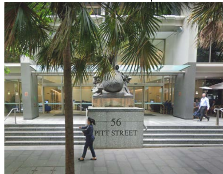
Existing Pitt and Bridge interface with Pitt St
