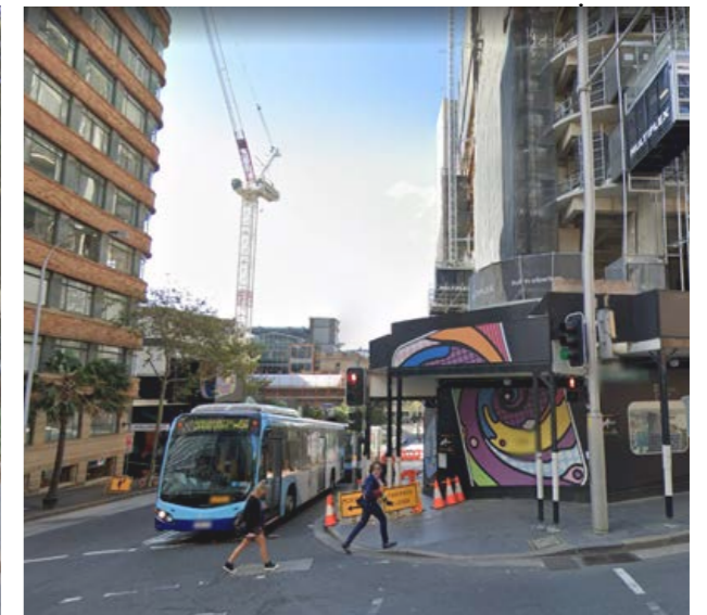
Quay Quarter under construction
